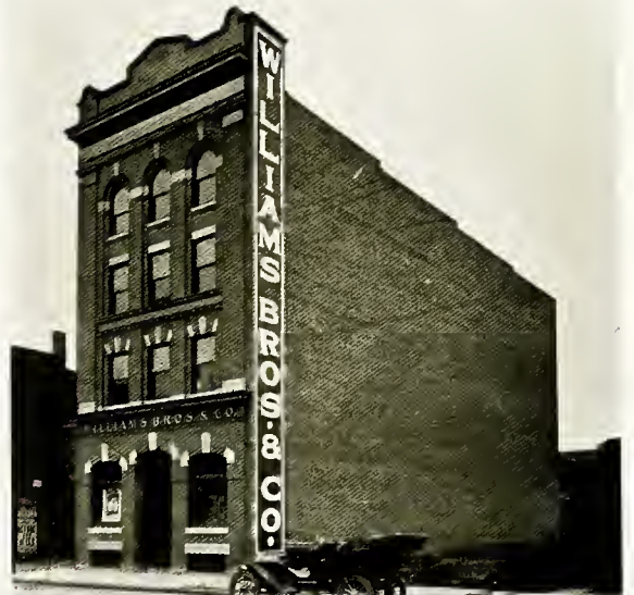
Williams Bros. & Co. Wholesale House South Pennsylvania Avenue
